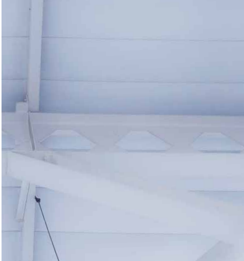
The Starlite® installation at Makro.
